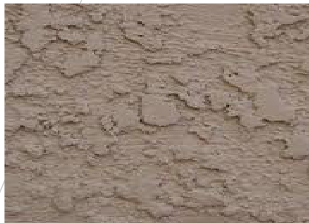
Figure 6: Example of troweled surface.
