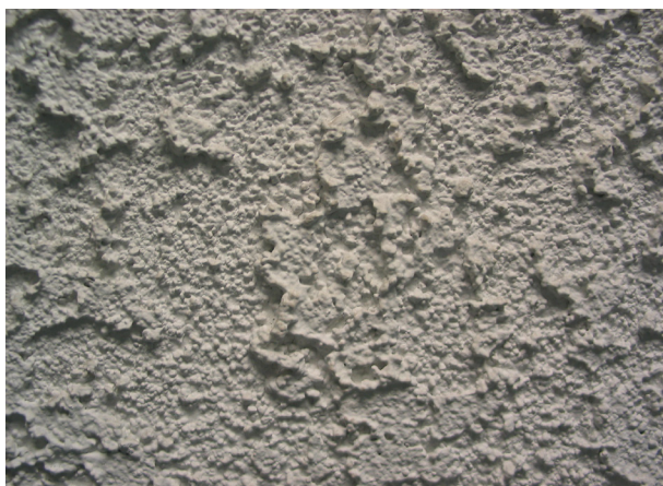
Figure 5: Example of stucco surface.
