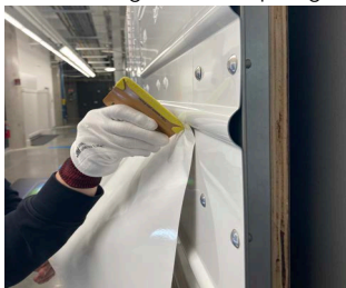
Figure 4. Squeegee the bottom of the corrugation.
