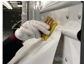
Figure 3. Squeegee the crown of the corrugation.
