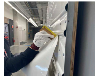
Figure 5. Squeegee the bottom of the corrugation.
